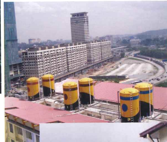
DBKL Bangsar Apartment, KL
